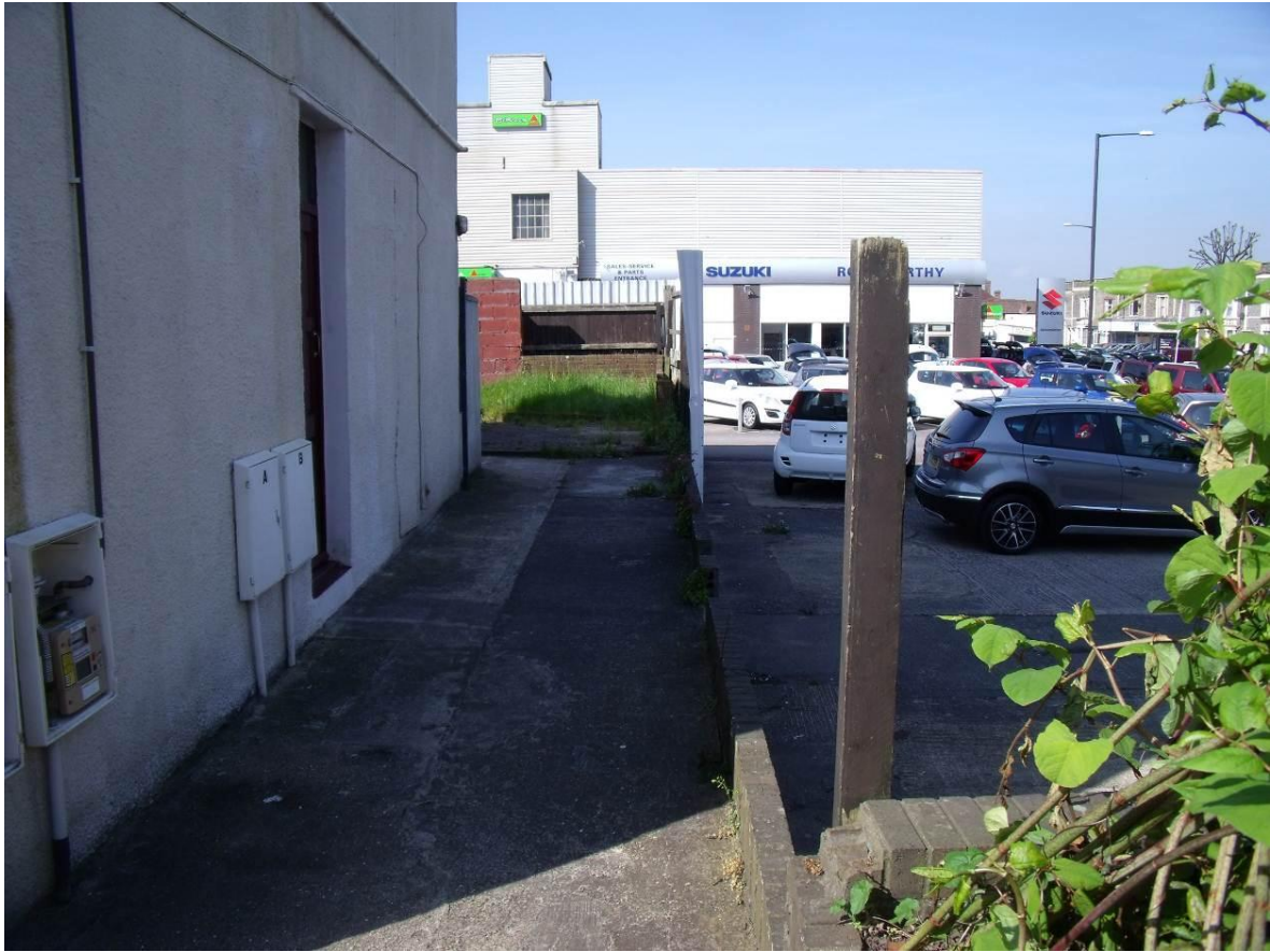
View into rear garden of adjacent property showing changes in level.
