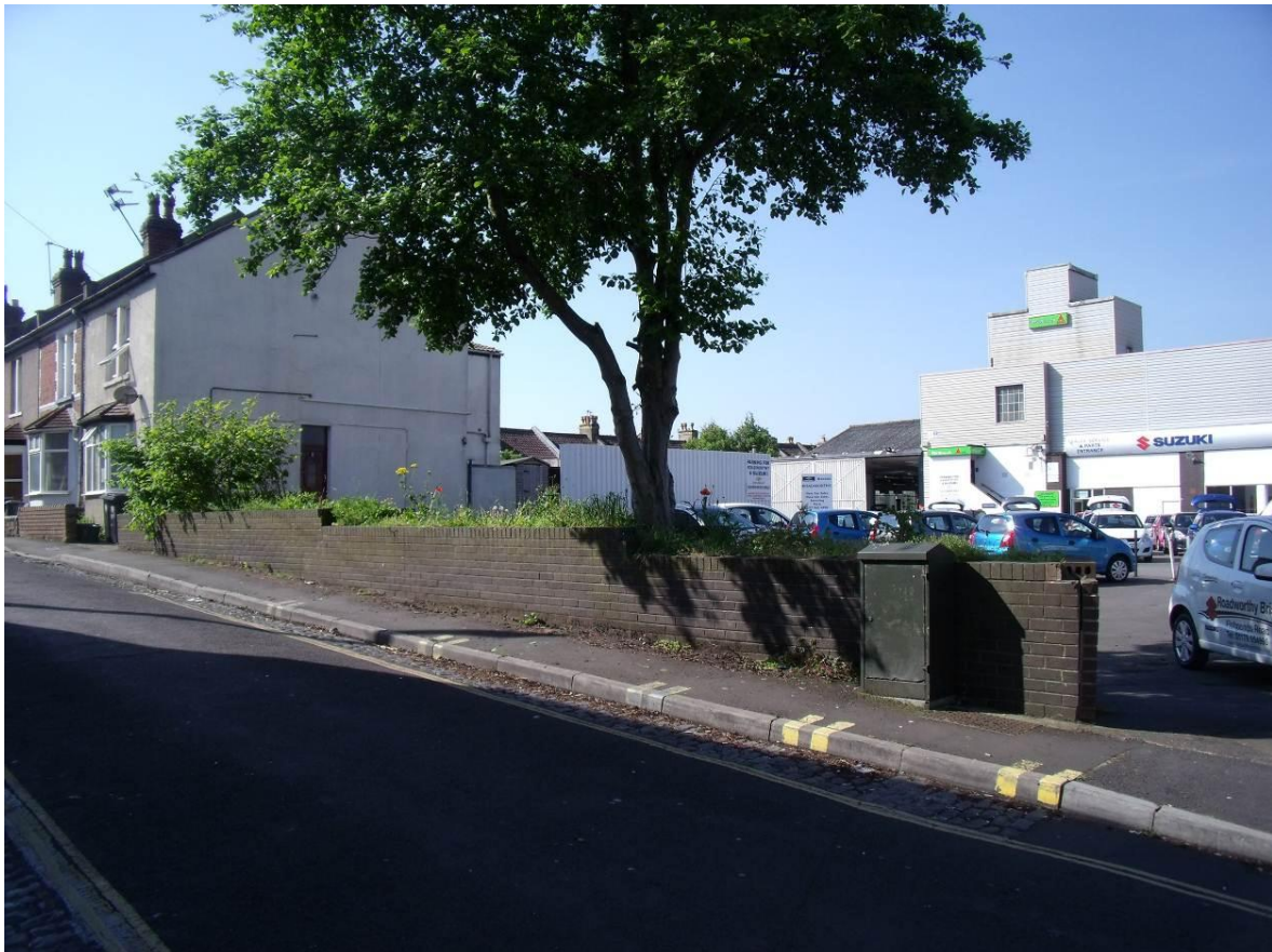
Existing retaining wall/raised planting bed to Ernestville Road
